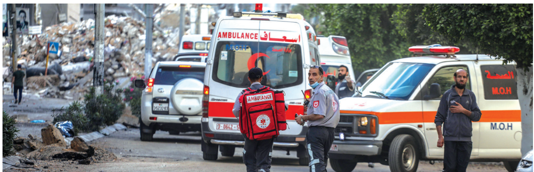
Damage to the Palestinian Ministry of Health building and Al-Rimal dispensary, Gaza City. (Credit: Mohammed Zaanoun)
